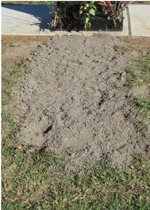
Stabilised grave covered in top soil in preparation for turf
